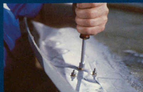
7) Through bolted deck hardware
